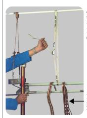
Add suspensions and adjust the section insulator height by value x according to Hogging Instruction on page 1. (if not known value = 70mm).
