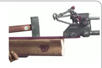
Buckling in contact wire can be repaired with hammer and straightening wood.
