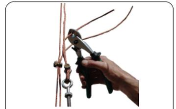
After complete hogging and fine adjustment cut the unnecessary dropper wire.
