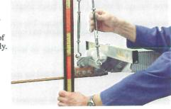
15. If available: Lock turnbuckles with a locking wire through the screw hole.
