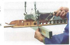
Readjust hangers before and after the insulator up to the guide arm clamps without affecting the adjustment of the section insulator height.
